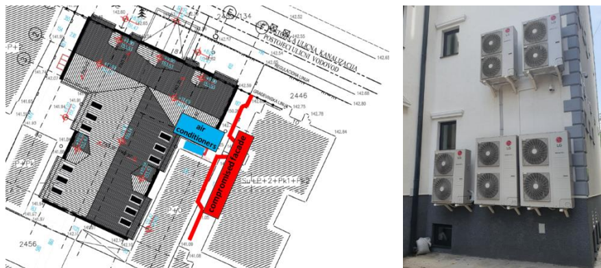
Fig. 1 General plan with the position of the office building where the air conditioners are located and affected endangered facades of the residential building (left) and a photo of the courtyard facade of the office building (right)
