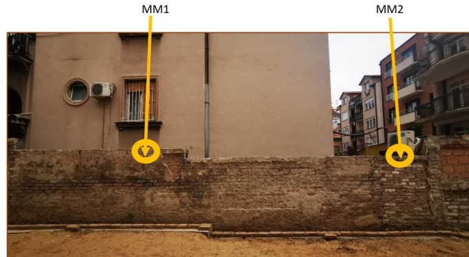
Fig. 5 Photograph of the wall separating the plot of the business building and the plot of the neighboring residential building; the positions of the measuring locations places are marked (view from the side of the office building)
