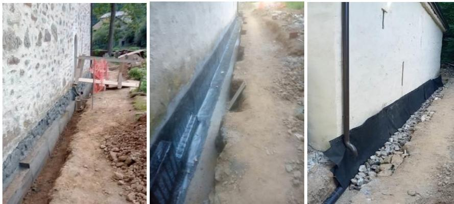
**Fig. 13** a) reconstruction of the plinth wall, b) hydro-isolation, c) drainage (Photo P.P.)
