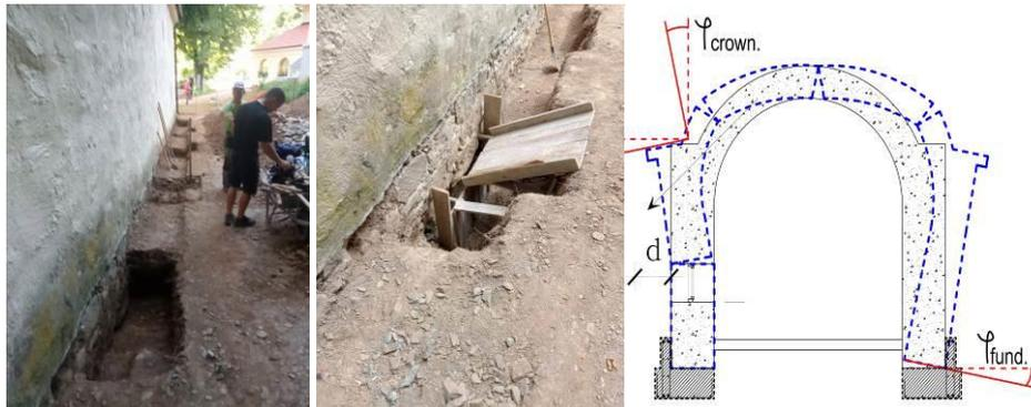
**Fig. 12** Foundation underpinning
