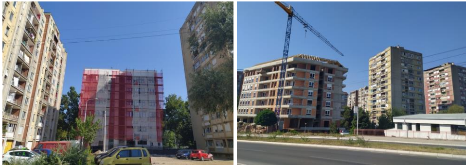
Fig. 3 Type of multi-family housing: New infill development - LHE Bulevar Nemanjića (source: authors)
