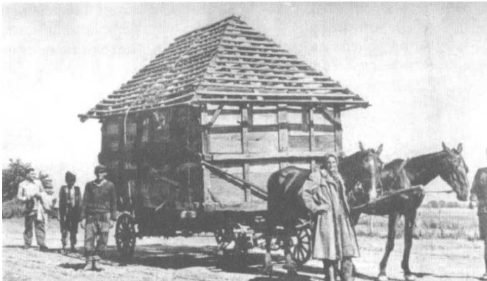
Fig. 2 Transport of a whole building
