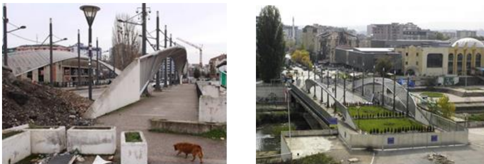
Fig. 4 The main bridge on the Ibar that connects North and South Kosovska Mitrovica, a bridge blocked by barricades recorded in March and as a green peace park in October 2014.
