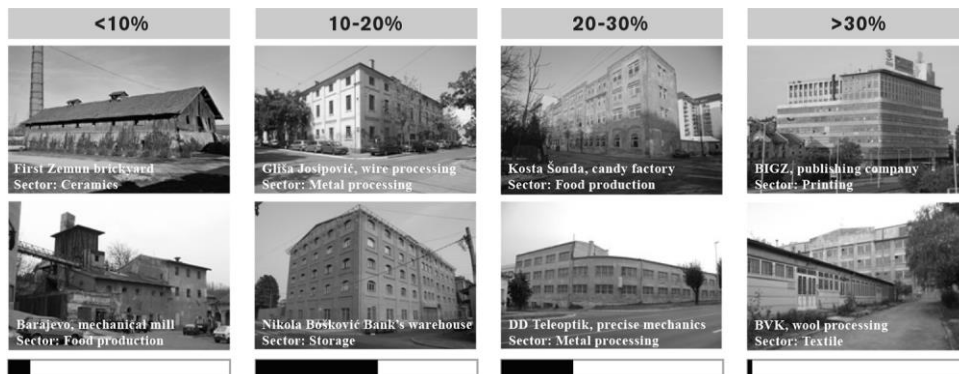
Fig. 1 Belgrade's industrial heritage - window to wall ratio categories (Sources: Images: Kulenović, 2010 and Museum of Yugoslav History [8])
