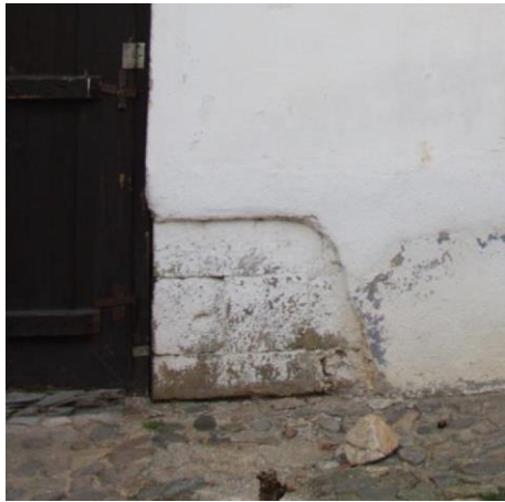
Fig. 7 Dressed stones, ground level
