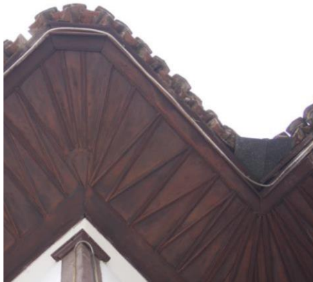
Fig. 9 Detail of eaves
