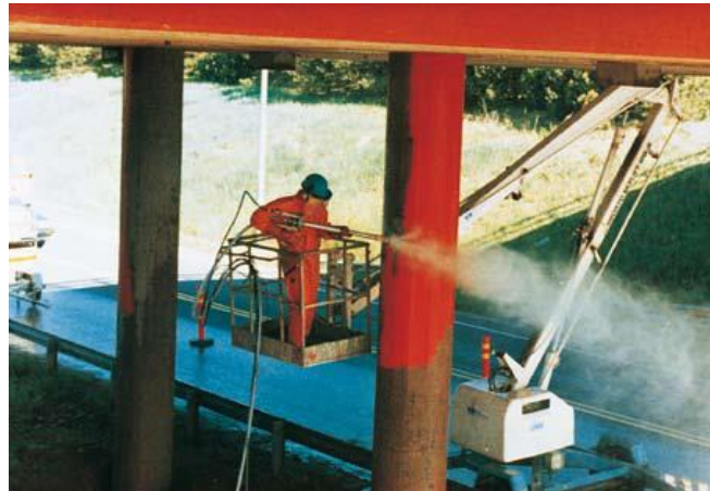
Fig. 8 Decoating of reinforced concrete with hand-held high-pressure water jet equipment
