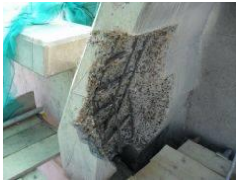
Fig. 6 Selective removal of deteriorated concrete
