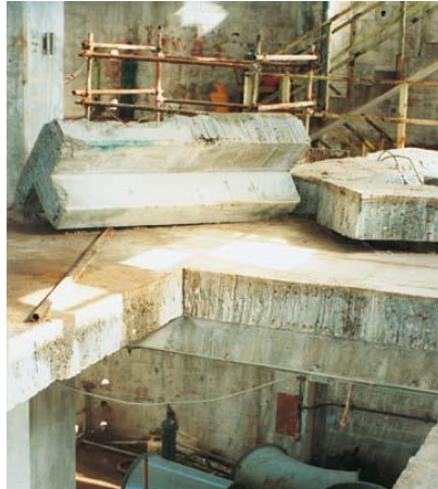
Fig. 9 Cutting of heavily reinforced concrete ceilings
