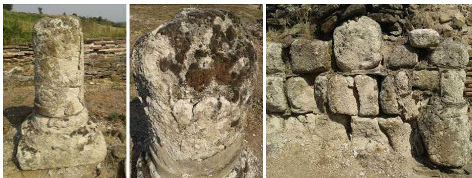
Fig. 6 Stone damage: flaking and crumbling (photo: A. Momčilović-Petronijević)
