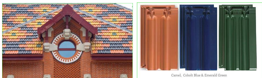
Fig. 12 "French tile or Marseille tile" by the French Gilardoni Brothers in 1850. Source [24]
