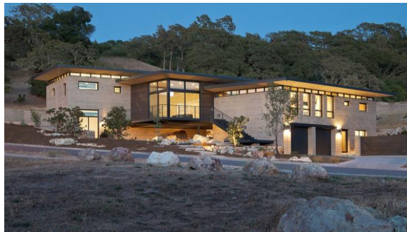
Fig. 11 House in Napa, California, architect Juliet Hsu 8
