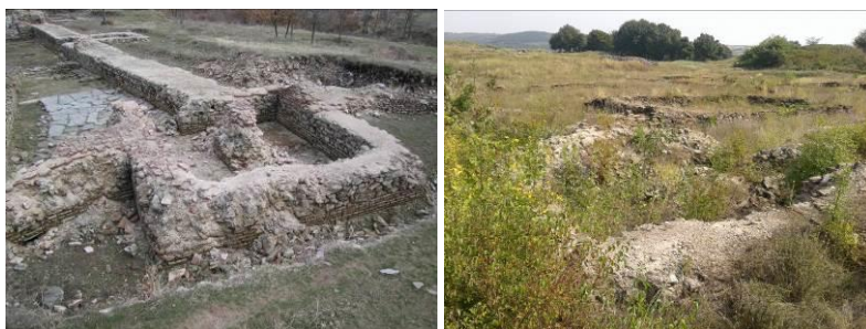
Fig. 4 Southwest corner tower of Lower Town within a span of several years (photo: A. Momčilović-Petronijević)
