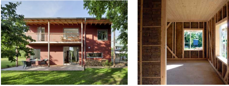
Fig. 3 The appearance of the basic structure and filling, the house during construction and after construction, Darmstadt, Germany, the project of the company "Schauer + Volhard" 2
