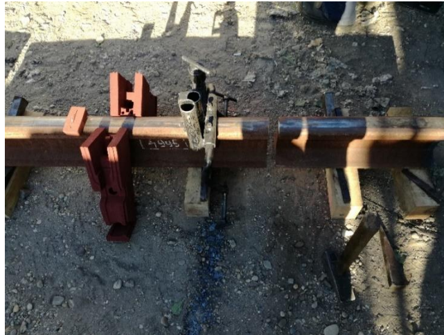
Fig. 1 Setting the rail ends as a function of the welding gap
