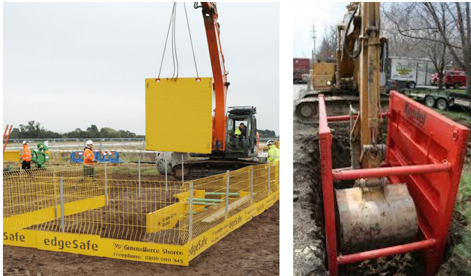
Fig. 8 Construction machinery excavation compliant with all the requirements
