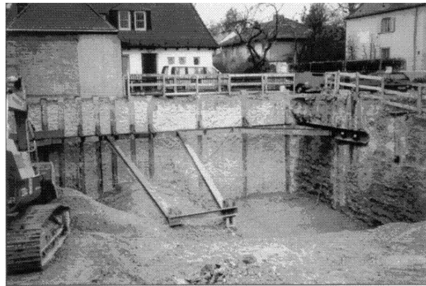
Fig. 7 Securing the retaining wall
