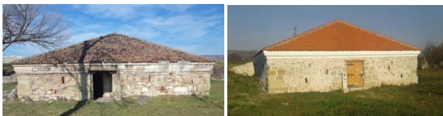
Fig. 8 Gunpowder magazine no 2 (left) and no 4 (right), Photo A.M.Petronijević.
