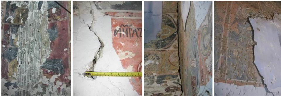
**Fig. 9** characteristic cracks between the vault and the transverse walls (photo. P.P.)
