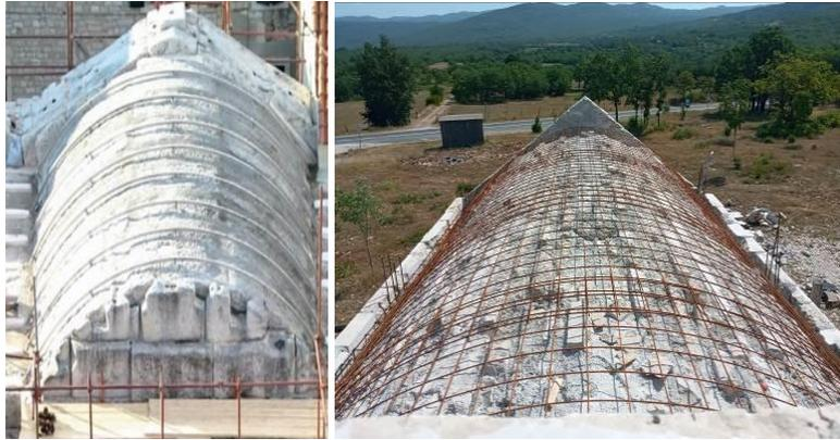
**Fig. 15** a) Reinforcement of the vault extrados with steel arches, b) masonry vault reinforcement with additional RC vault (photo: P.P.)
