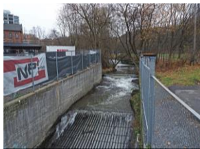
A. Culvert of Alna at Kvaernerfossene.
