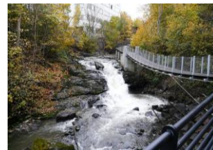
C. Suspension bridge along Alna, Svartdalen.
