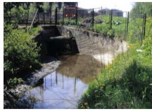
A. Culvert of Hovinbekken under the subway at Risløkka. https://hovinbekken.org/vandring/
