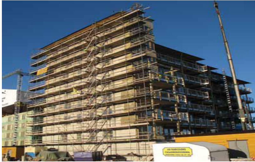
Fig. 4 Växjö, Sweden/2008, Residential: 1+7 stories (last as duplex), 4 buildings, 10,700 m 2 , CLT 4,800 m 3 ( KLH catalogues http://www.klh.at ).
