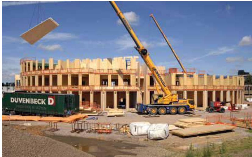
Fig. 6 Norwich open academy: 3 stories, UK/ 2010, floor area 9500 m 2 , CLT 3600 m 3 , 18 weeks (KLH catalogues http://www.klh.at ).
