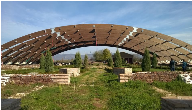
Fig. 5 Mediana, shelter in construction phase
