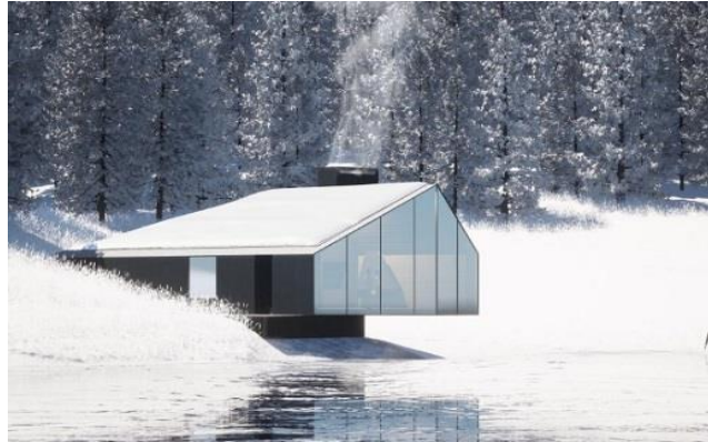
Fig. 12 The Experimental Shelter, Italy. (Source: https://www.archdaily.com )
