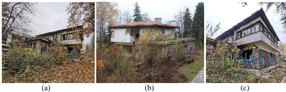
Fig. 9 (a) (b) (c) Condition before demolition of Crni vrh urban villa. (Source: author's archive, 2020)
