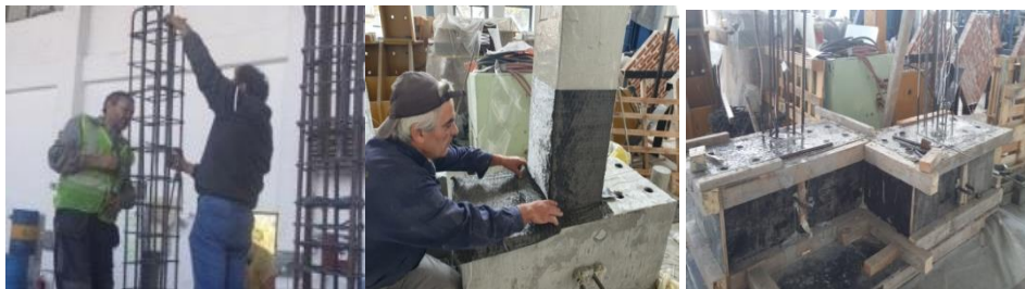
Fig. 1 Construction of the column models for experimental tests and Photos taken during application of FRP on the mode
