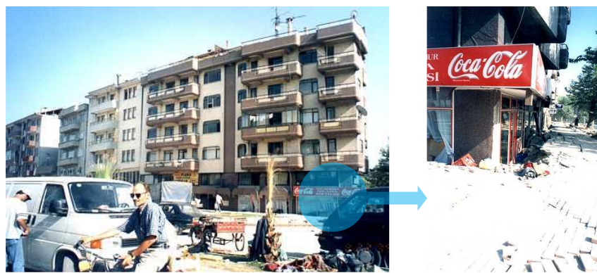
Fig. 30 Settlement due to soil failure – Kocaeli (Turkey) earthquake (1999)
