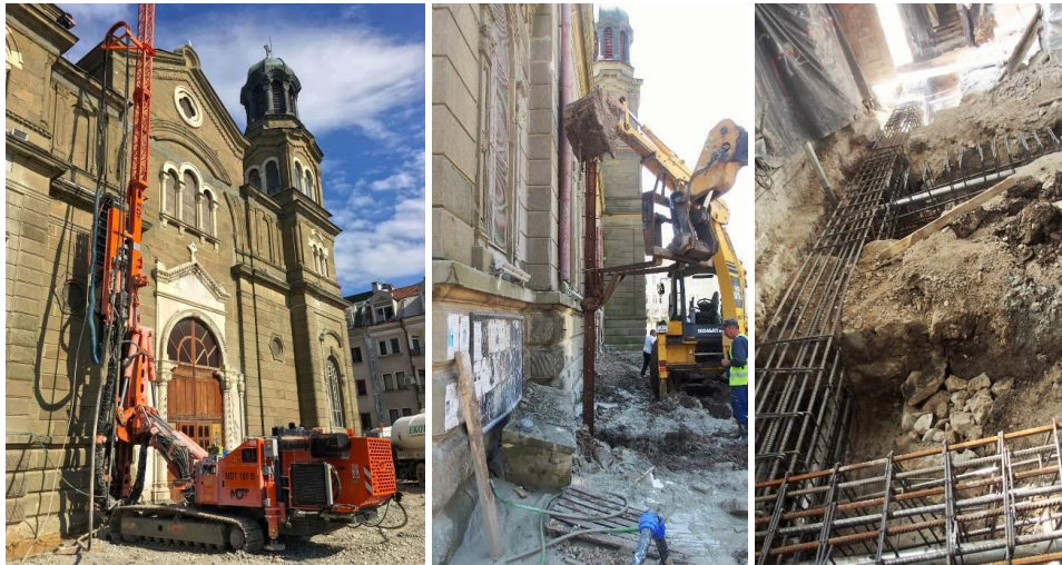
Fig. 14 Execution process – rescuing the “St. Cyril and St. Methodius” cathedral
