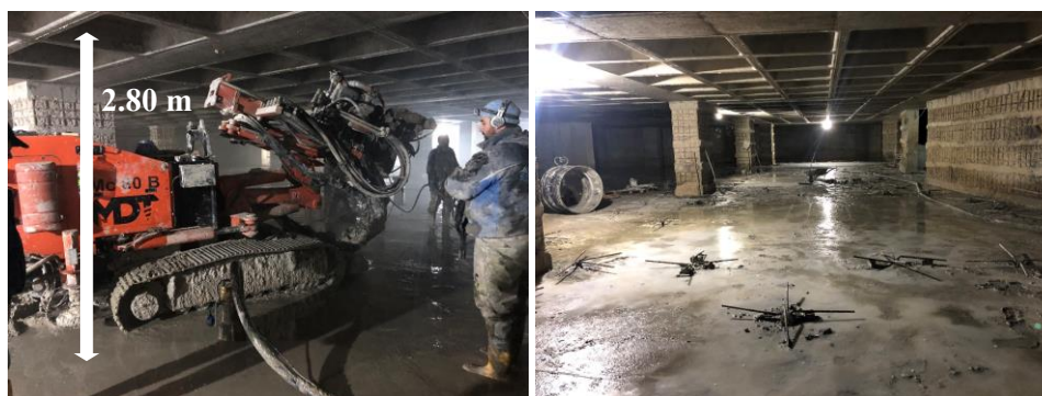
Fig. 12 Execution of the strengthening measures
