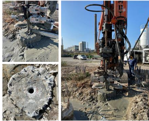
Fig. 16 Execution process –strengthening of piles by the jet grouting technique
