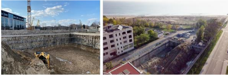
Fig. 8 Excavation execution process
