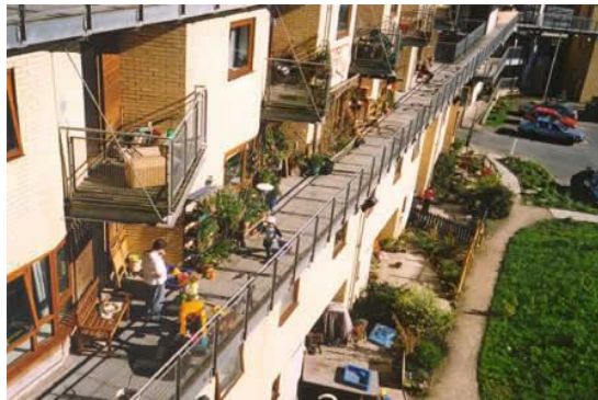
Fig. 2 Homes for Change, Manchester, UK, MBLA Architects+Urbanists
