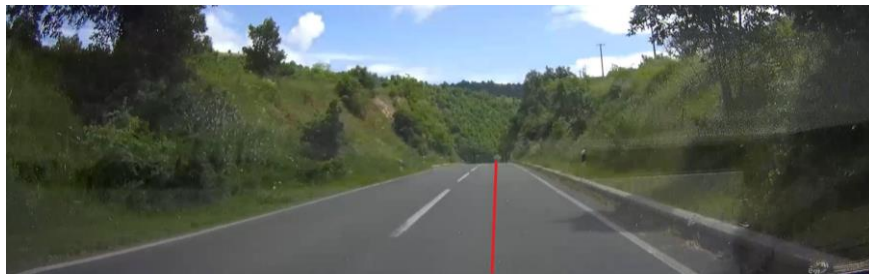
Fig. 5 Vertical SSD at speed of V=70\text{km/h} and a visible beam of Pz=90\text{m} , section: A3 Prevalec – Kamenica
