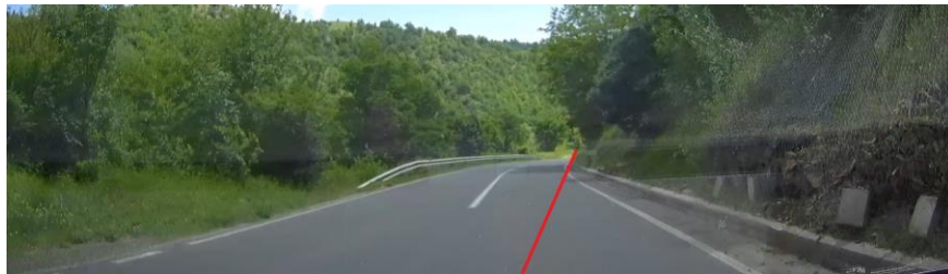
Fig. 4 Horizontal SSD at speed of V=70\text{km/h} and a visible beam of Pz=90\text{m} , section: A3 Prevalec – Kamenica
