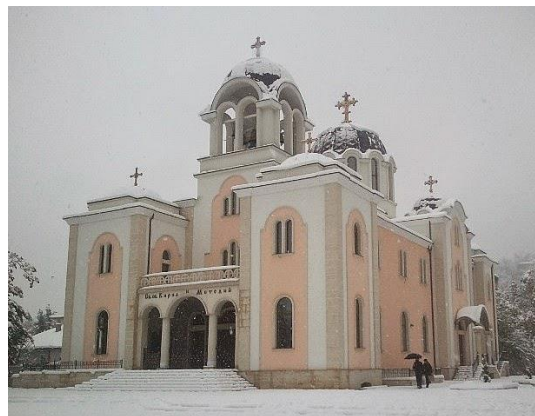
Fig. 1 St. Cyril and Methodius Church in Lovech (2014) – architect Ts. Kovacheva (Source: https://nglas.wordpress.com )
