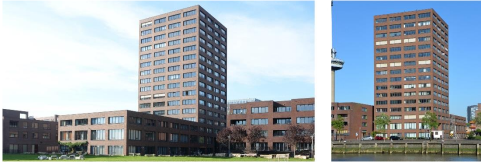
Fig. 7 De Ruyter residential building (Rotterdam, St. Jobskade; designed by F. Van Dongen), built in 2003, was first named Big Foot for its configuration in the form of a tower with distinct low block volume. The low block was created to accommodate additional dwelling units, outside storage areas and enough space for two-level underground parking garage. Photos by Mirko Todorović, 2015.
