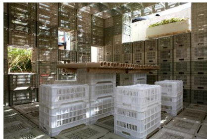
Fig. 6 Emergency shelter with plastic crates + ties for Syrian refugees, LAU 2014. Instructor Ricard Douzjian
