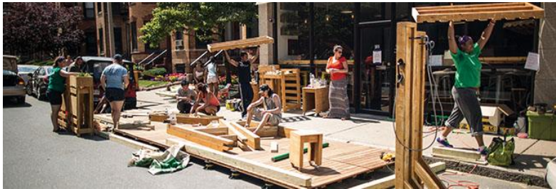
Fig. 4 Installation of Parkolation project Gateway initiative Spring 2014 Boston Architectural College
