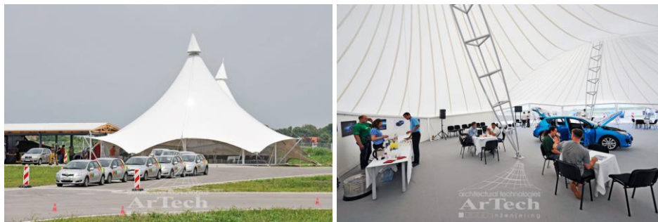
Fig. 1 NAVAK in Serbia, constructed by ArTech, exterior and interior view
