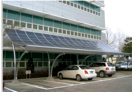
Fig. 5 An example of a building integrated photovoltaic system
