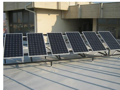
Fig. 4 Rooftop construction – solar plant in the city of Niš
