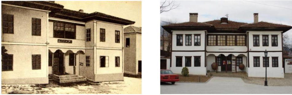
Fig. 2, 3 View of the entry façade of the grammar school prior to its moving out, around 1930, archive photo and in 2012, photo Z. Radosavljevic Kiki
