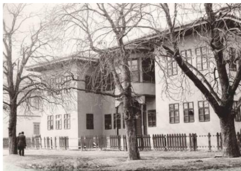
Fig. 9 East façade of the Haremluk
