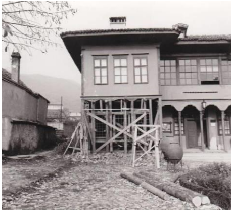
Fig. 10 A part of the Selamluk south facade 1972.
