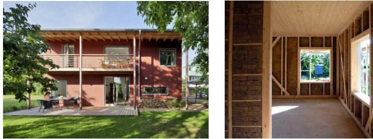
Fig. 3 The appearance of the basic structure and filling, the house during construction and after construction, Darmstadt, Germany, the project of the company "Schauer + Volhard" 2
