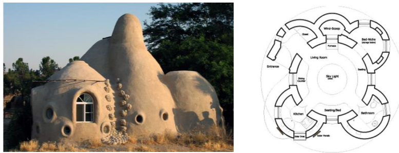
Fig. 8 Construction of ceramic houses in America, architect Nader Khalili 6
