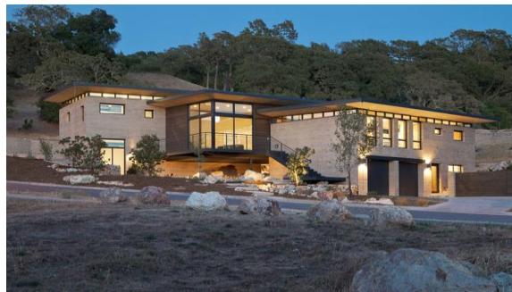
Fig. 11 House in Napa, California, architect Juliet Hsu 8
