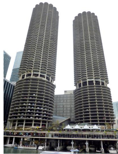
The garage of Marina City towers, architect HENN Bertrand Goldberg, Chicago, Illinois 1964
