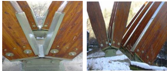
Fig. 4 Details of supports-correct solution
