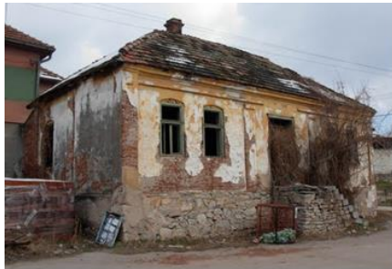
Fig. 4 An abandoned house in the village Donji Matejevac (source: authors)
