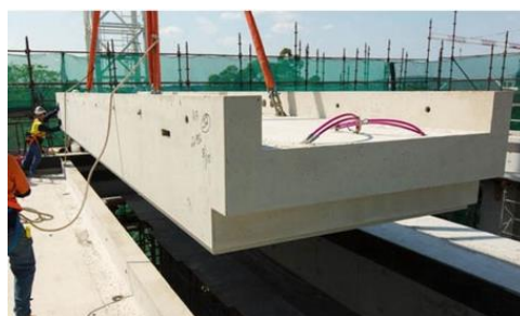
Fig. 8 Queensland's University building [16]. Fig. 9 Construction of floor [17].
