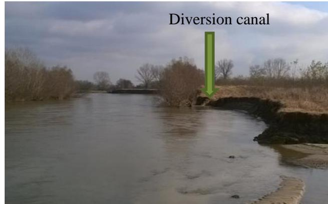
**Fig. 4** River bed erosion and collapsed water intake
