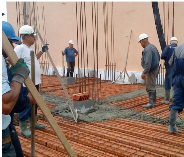
Fig. 5 Concreting of "fert" ceiling (photo by the author of the paper)
