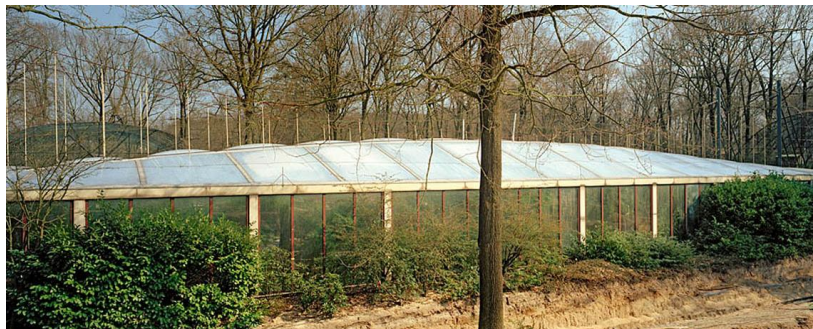
Fig. 1. The first structure clad by ETFE single layer at Burgers Zoo [3]
