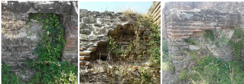
Fig. 9 Open caverns in the massive fortification walls (photo. A.M.Petronijević)
