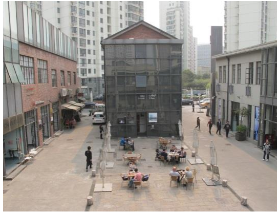
Fig 2 50 Moganshan Road in Shanghai, China: cultural and creative cluster, area with café in a renovated old industrial building.
