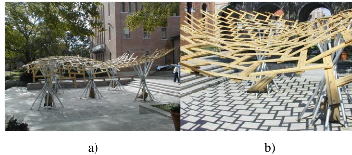
Fig. 6 Pavilion of the Forest Park: the whole structure 6 (Source: Gherardini et al. 2017)
