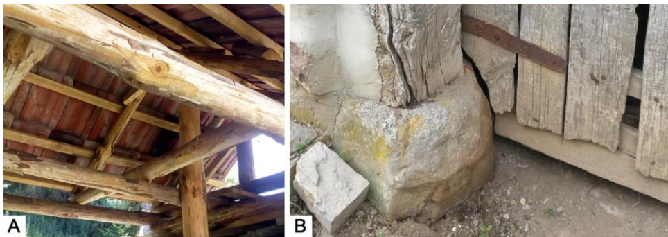
Fig. 8 Timber post resting on a stone footing (photo I. Đorđević)
