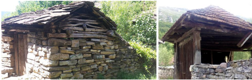
Fig. 7 Extended roofs near the gates with a storage space (photo I. Đorđević)
