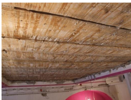
Fig. 5 Photograph of the ceiling made of timber half-cylinders on the ground floor of the former hotel “Hungaria” (photograph author: Viktorija Aladžić)
