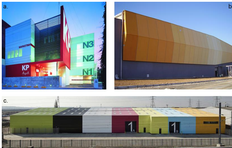
Fig. 1 a) KP Alazraki Corporate Building, Mexico (ph. Mito Covarrubias ); b) Stoby Winery, North Macedonia (ph. credits: Aleksandar Radevski & Viktorija Stavrik ); c) Wildspace, United Kingdom (ph. Tim Crocker )
