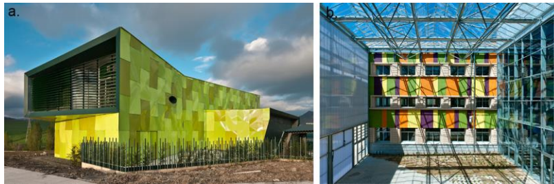
Fig. 4 a) Urban Solid Waste Collection Central, Spain (ph. credits: Vaillo + Irigaray ). b) Pccital Gardeny, Spain (ph. Jordi V. Pou )
