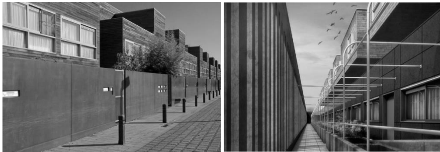
Fig. 2 Hollainhof social housing (1998), Gent, Belgium / Neutelings – Riedijk
