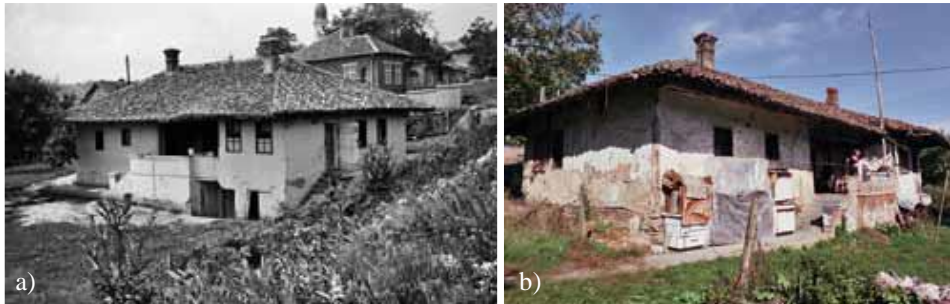
Fig. 4 Vljaković's house in Grocka: a) Appearance of the house in 1972 b) Current condition (Sources: M. Dedić, S. Negovanović)
