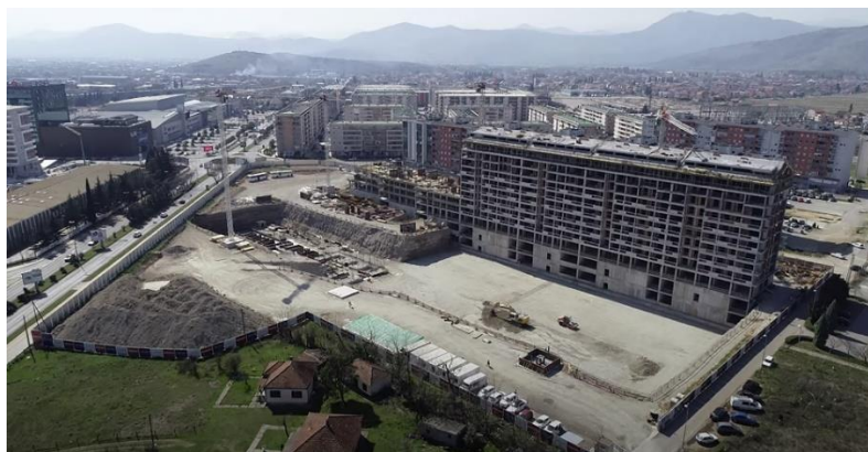
Fig. 6 “Master Quart” – under construction (Source: https://www.youtube.com/watch?v=Odos3utXmTI )
