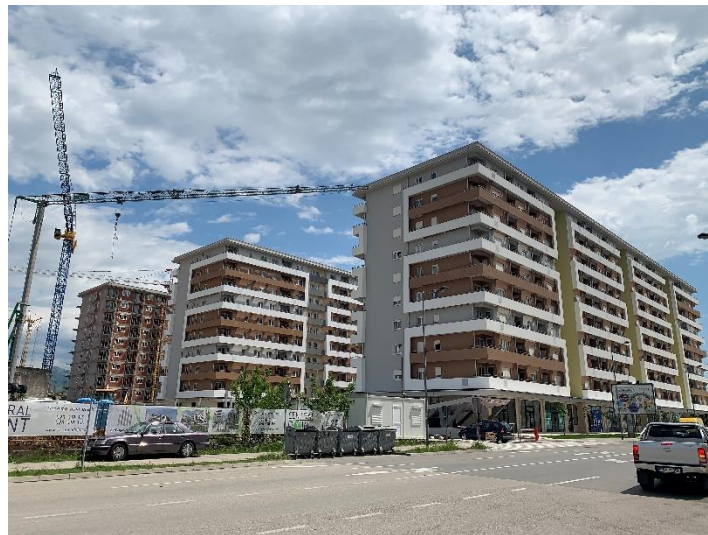
Fig. 5 “Central Point” – under construction (Source: personal collection)
