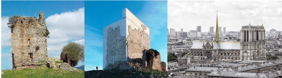
Fig. 1 a) Castle of Matrera before and after the restoration, b) One of the proposals for Notre Dame's reconstruction
