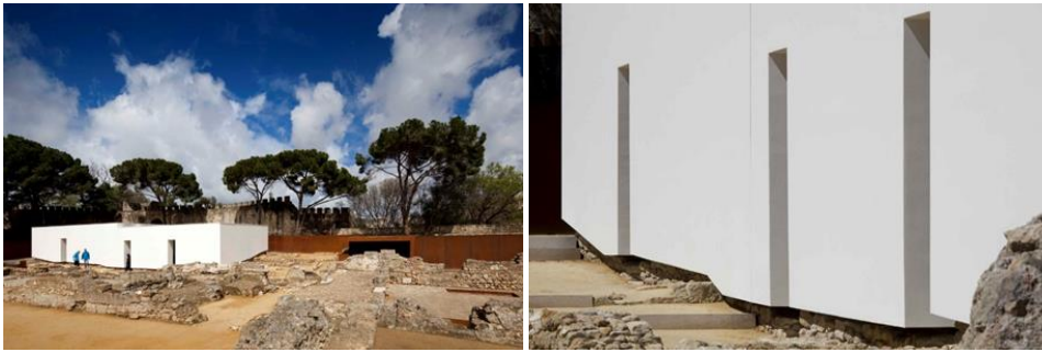
Fig. 6 A hovering protecting new structure
