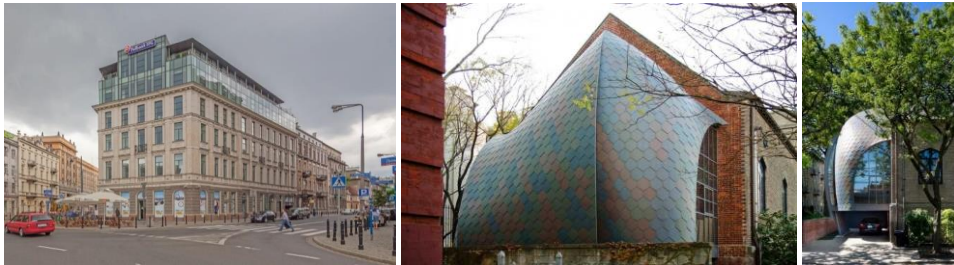
Fig. 9 a) The extension of the Pawłowicz House, b) and c) Studio extension of a church in Hoboken
