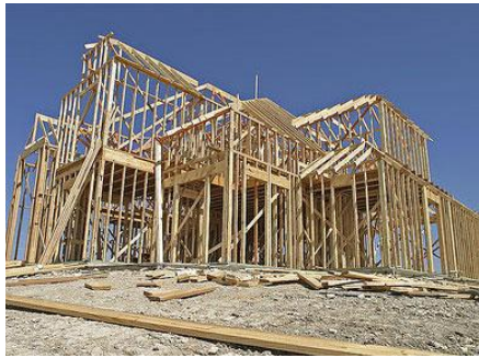
Lightweight timber construction
