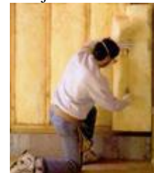
Fiberglass installation
