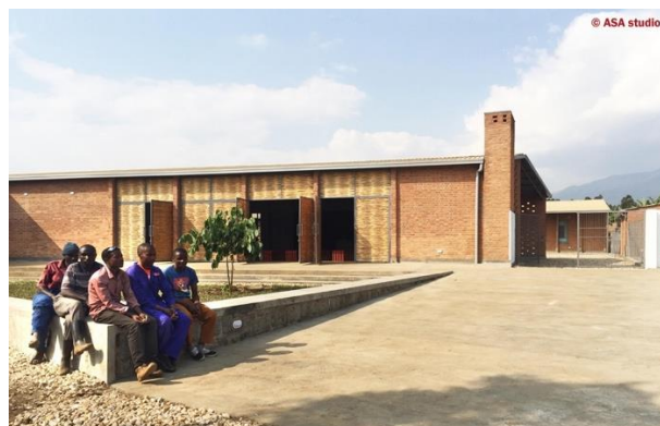
Fig. 3 Health Center and public space in front of the building © ASA studio
