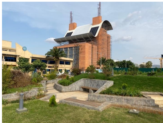
Fig. 1 I&M Bank HQ under construction © Ilija Gubić
