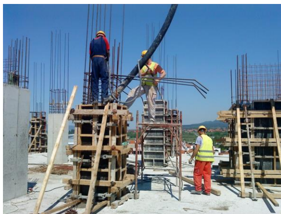
Fig. 2 Concreting of reinforced concrete columns (photo by the author of the paper)
