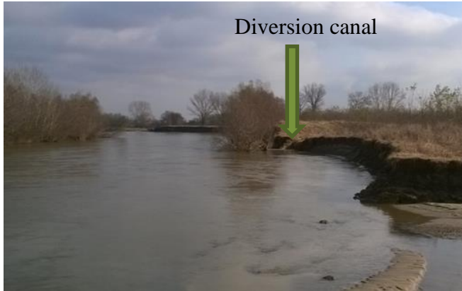
Fig. 4 River bed erosion and collapsed water intake
