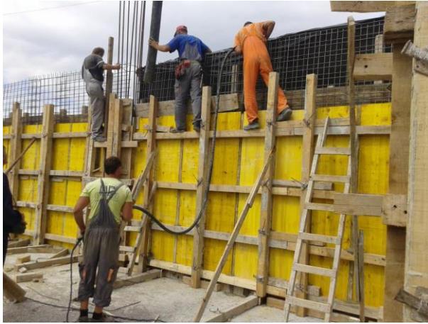
Fig. 3 Concreting of reinforced concrete walls (photo by the author of the paper)
