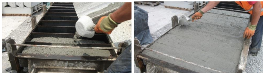
Fig. 5 Production of curbs made of SCC with CRT glass admixture
